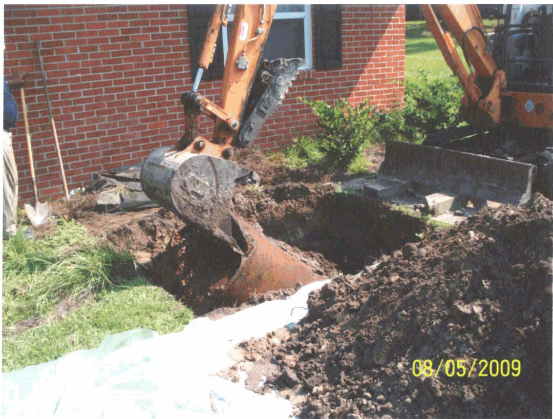
Picture 2: UST 1442Dove-2 during removal from excavation.
