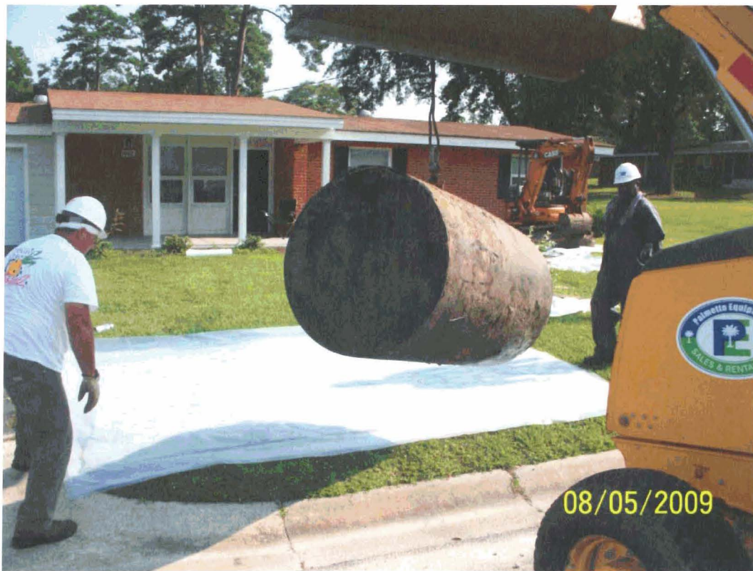
Picture 2: UST 1442Dove-1 during removal and containment in poly.
